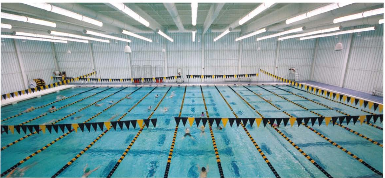
The main feature of the athletic center is the natatorium (above), which houses a competition-regulation swimming pool. The pool is lit with a light-pipe system that uses 1,000W metal halide lamps to provide the required 50-footcandle-level of glare-free illumination on the water surface. Metal halide downlights illuminate the surrounding deck areas.
