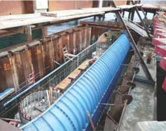
Stage 1 construction utilizing reusable steel footing form. Photo: K. Pope, T.Y. Lin International.
