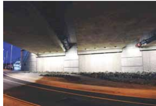
The Cypress Avenue Bridge in Redding, Calif., uses metal halide fixtures to illuminate the textured, vertical surface, eliminating shadows and welcoming pedestrians to traverse the area beneath the bridge.
