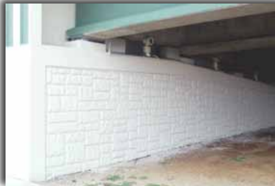
At Biloxi Bay Bridge, the aesthetic lighting design seeks to highlight the concrete girder pattern under the bridge by placing narrow beam, metal halide floodlights between the girders.
